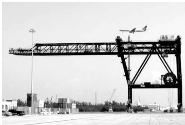
Fig.8: Low profile container crane.
