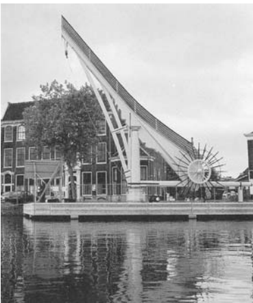
Fig.3: Wooden slewing crane.
