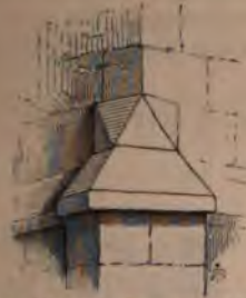
Capping of Tower Buttresses, St. Wendron.
