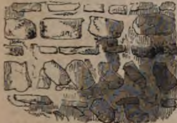
1. Gundulf's Tower at Malling, Kent, c. 1080.
