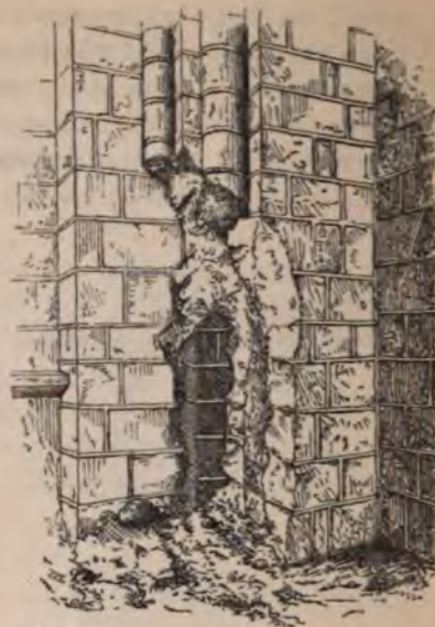
6. Masonry of the First Period, partly concealed by that of the Second Period.
