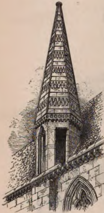
27. Top of Stair-turret with Spire, forming part of the building called the Tribunal.
