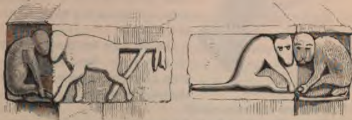
Gable Corbels of Porch, St. Germoe.
